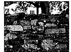
Clear away brush and debris, and place stones tightly together.
